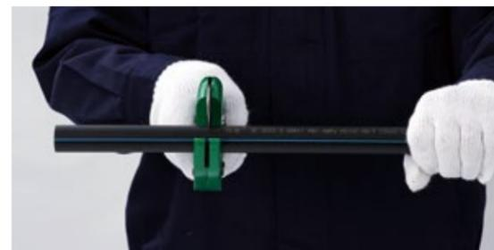
2. Scrape the outside of the pipe spigot to remove the outside layer from the pipe. Do not scrape the inside of the sockets.
