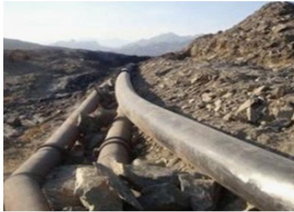
PE pipe is widely used in above ground applications, particularly in demanding conditions typical of mining and rural regions.
